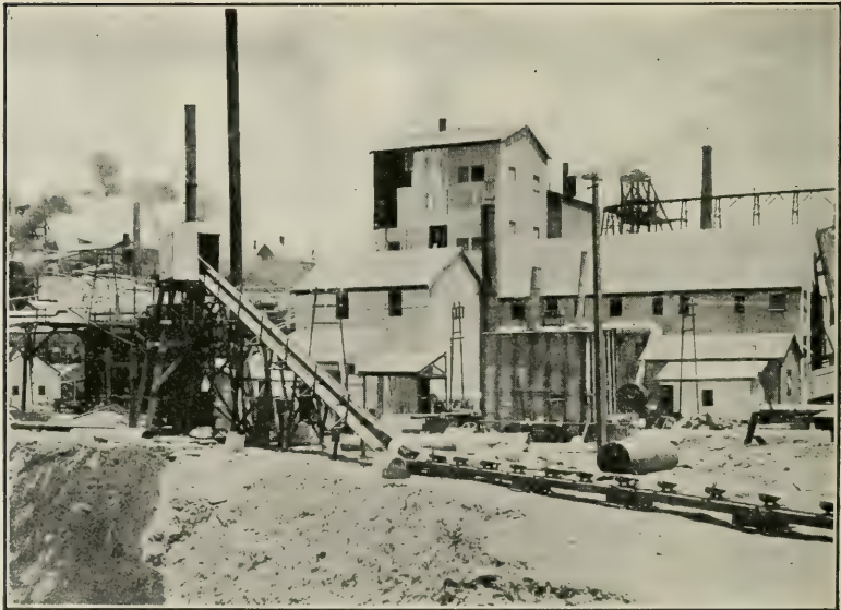
FIG. 75.—CONVEYOR FROM DUMP, PLANT NO. 2, SULPHIDE CORPORATION.
